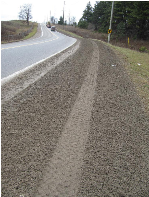
Figure 1 - Tire mark of road grader on freshly re-graded gravel shoulder
